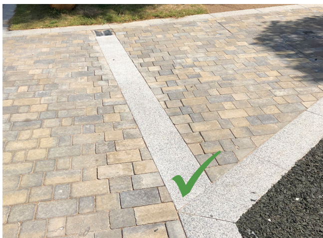
Dish gully replacement - Chesnut Road
