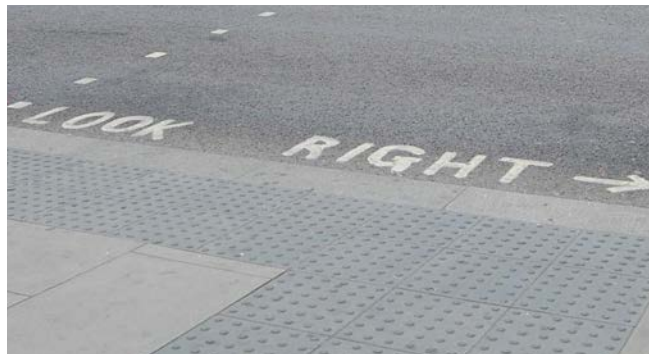
Tactile paving - High Road (A10)
