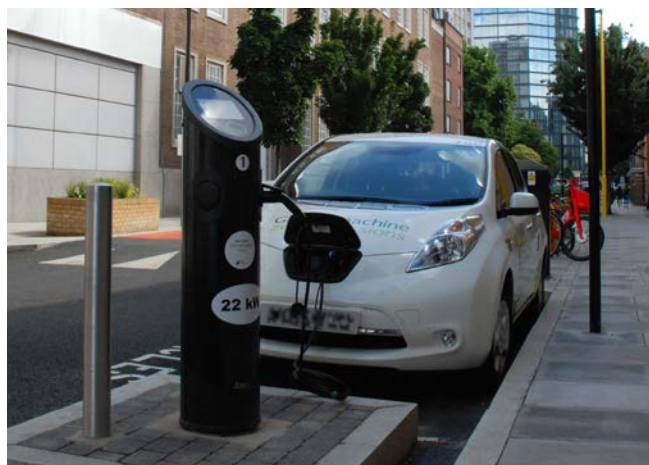
Electric charging point - Moreland Rd, Islington
