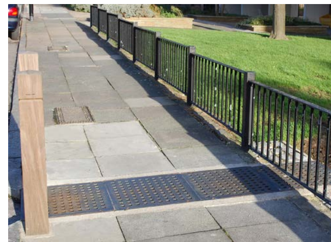
Drainage gully - Boyton Road
