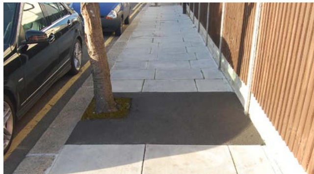
Alternative footway material – Ranelagh Road
