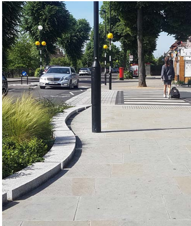
Footway and crossing - Dalgarno Gardens
