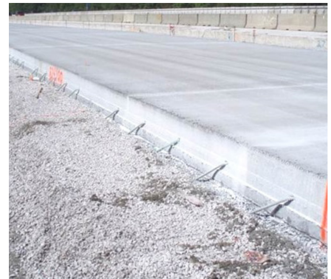
Reinforced concrete under the paving layer
