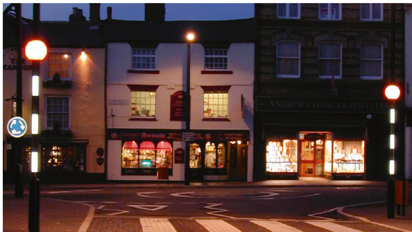
Pedestrian crossing control unit
