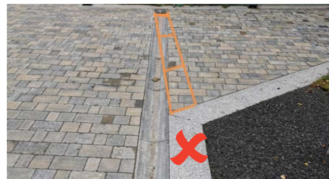
Dish gully replacement - Chesnut Road, Tottenham
